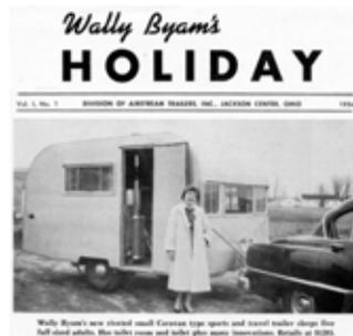
Holiday trailers had a "canned ham" shape with flat sides, a riveted aluminum skin, and a wood lined interior. Most Holidays were 15' single axle models, but a few 21' tandem axle models were also made for 1955. The single axle Holiday floor plan was very similar to that of the 1955-57 16' Airstream Bubble.
